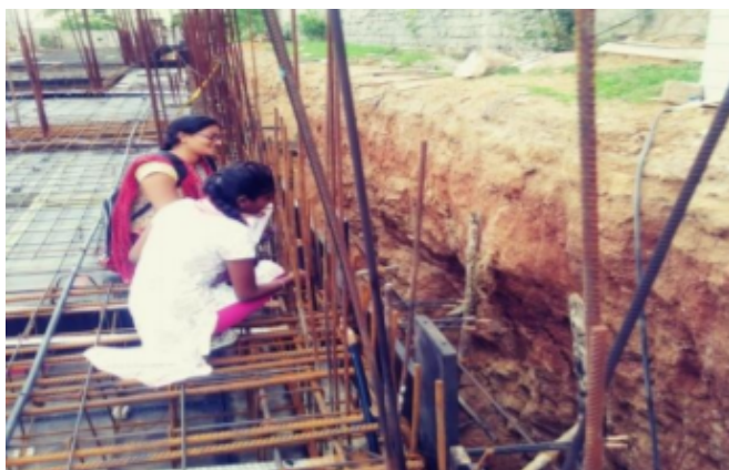
REINFORCEMENT OF RESIDENTIAL BUILDING
