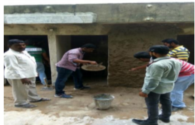
PLASTERING WORK DONE BY STUDENTS
